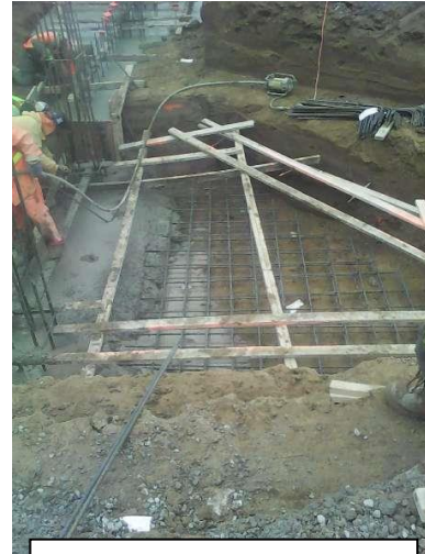
Rebar Ice Melting Pit Slab A-line
