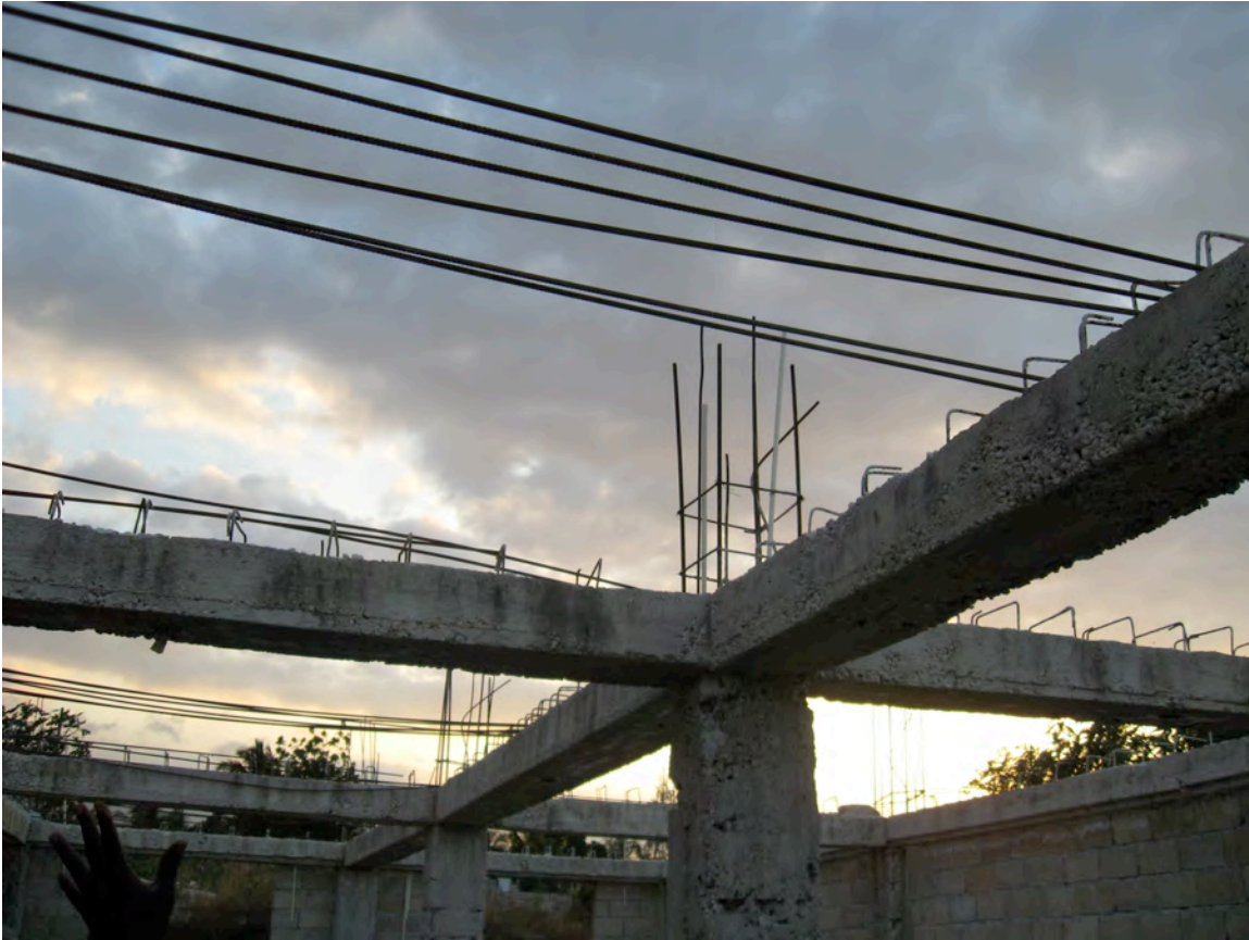
At another building site the first floor has been completed and rebar and concrete framing is in place to begin work on the second floor.
