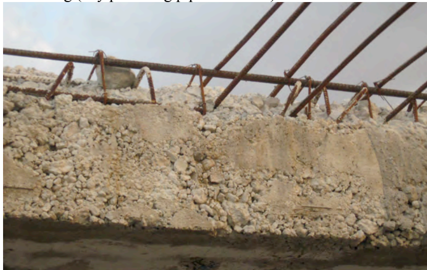
This photograph shows the concrete-imbedded rebar for the first floor ceiling at another building site.
