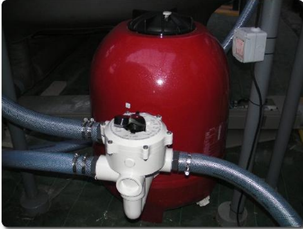
Mechanical sand filter
