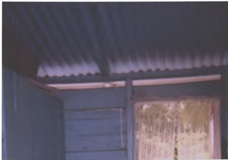
Figure 17a: Interior View of Opening between Roof and Wall. This narrow gap facilitates cooling of interior spaces as well as the roof.
