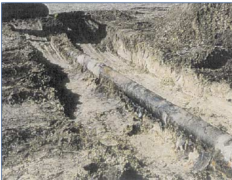
Damaged Pipeline Section (Photo Courtesy of Williams Pipe Line Company)
