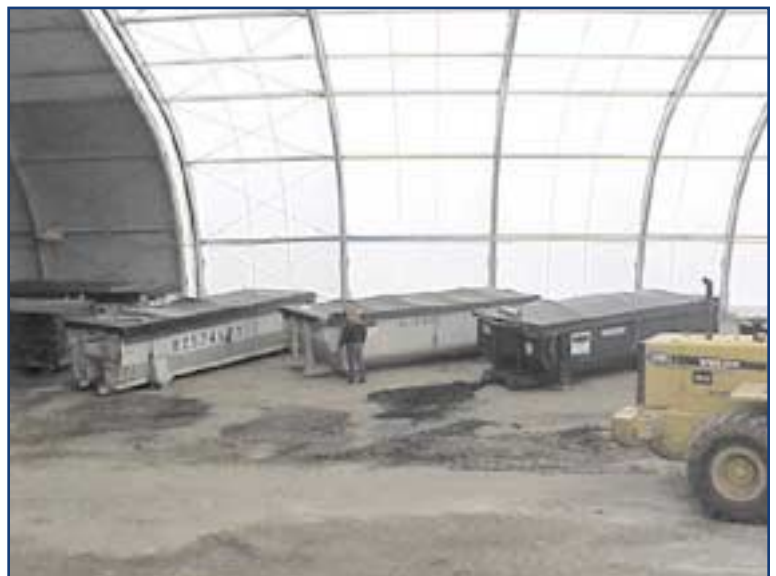
Excavated Material in Lined Containers Located Inside Containment Dome Awaiting Off-site Disposal
