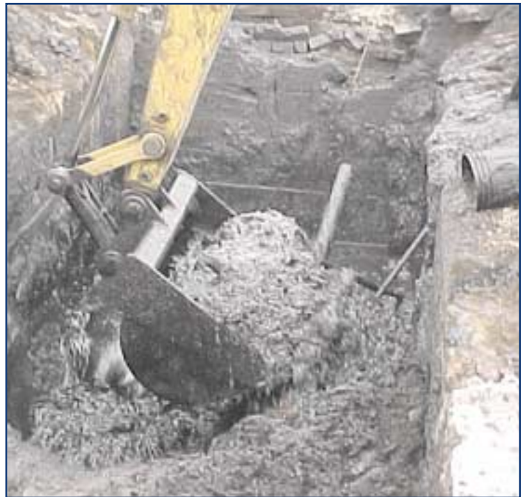
Removing Waste from a Tar Well (Beardstown)
