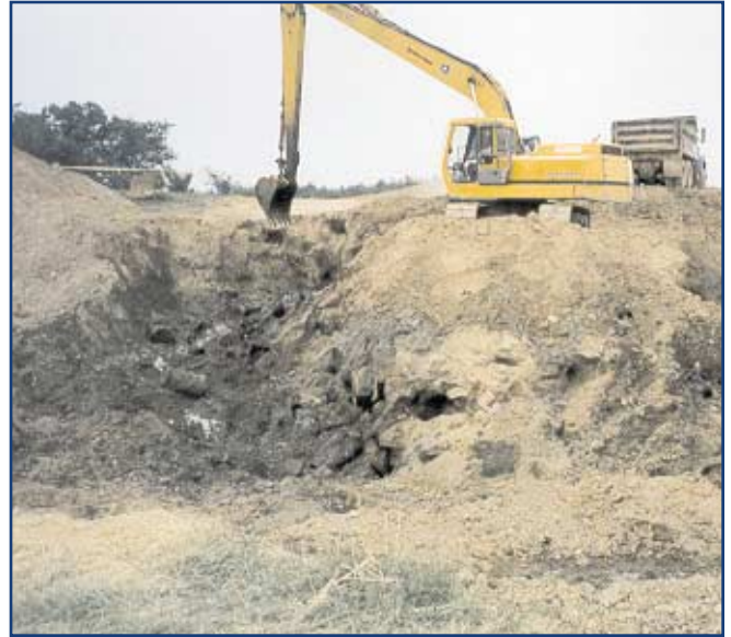
Removal of drums and contaminated soils (Photo Courtesy of Lonza, Inc.)
